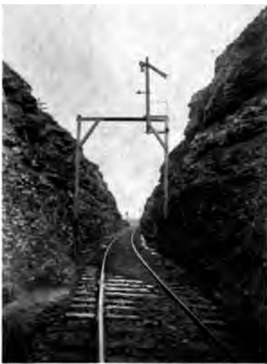
ENTRANCE TO KING'S MOUNTAIN TUNNEL. Altitude of hill above tunnel, 1287 feet. Length of tunnel, 3984 feet.
